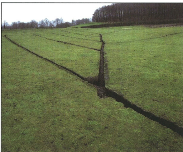
Pipe drains being installed using a tractor mounted drainage trencher (left). Using a dedicated drainage trencher produces clean trenches (right) and minimum disruption to the playing surfaces
