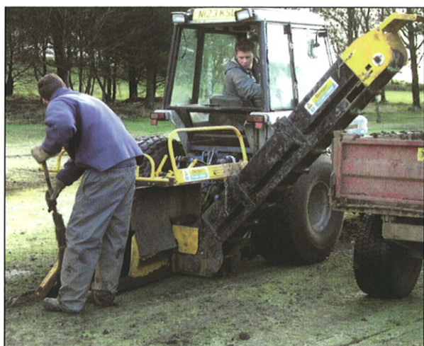
Pipe drains being installed using a tractor mounted drainage trencher (left). Using a dedicated drainage trencher produces clean trenches (right) and minimum disruption to the playing surfaces
