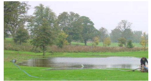
Area of frequent flooding
