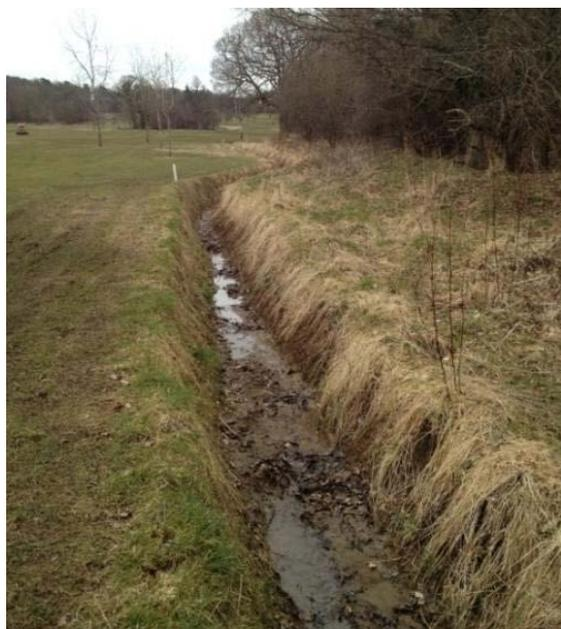
*Large trenches along the side of fairways allowing surface water to be collected and moved away from playing surfaces*
