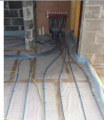
Underfloor heating system during installation
